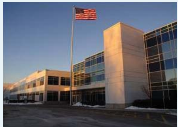
Above: Blue Cod's Class A co-location facility, Navisite, located in Andover, MA.
